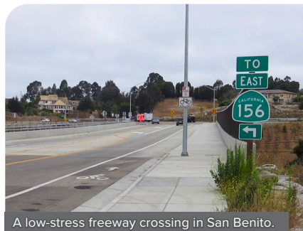
A low-stress freeway crossing in San Benito.
