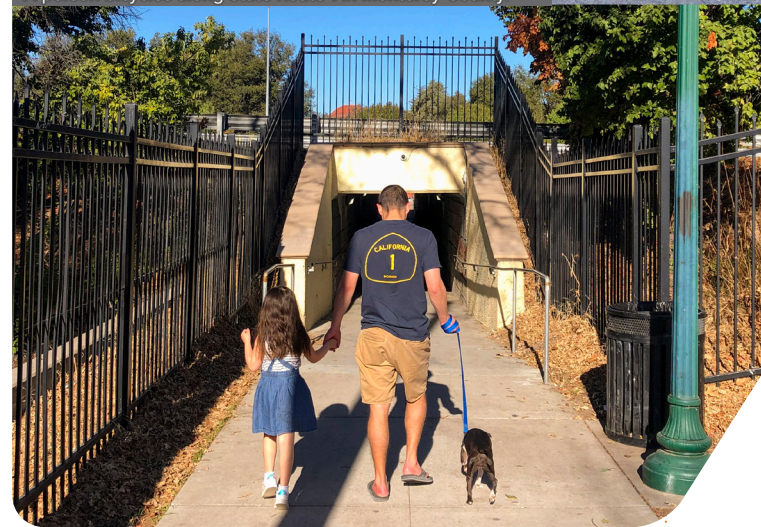
A US 101 freeway undercrossing in Atascadero.
