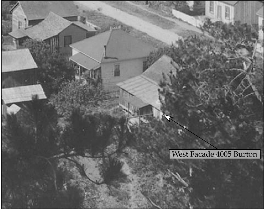
Figure 9: Back side of 4005 Burton Street Between 1910 & 1913
