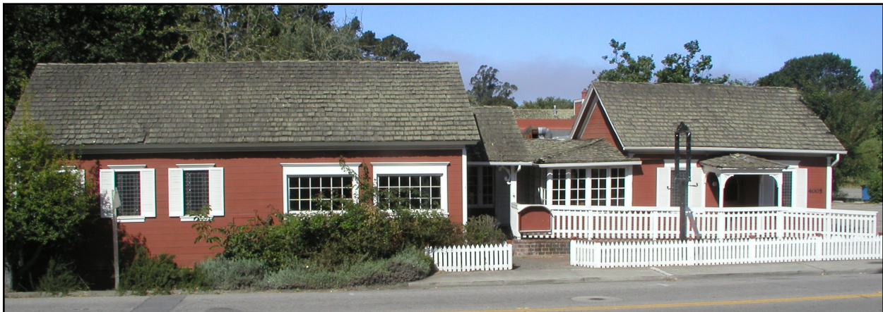
Figure 12: East Facade (August 2012)
