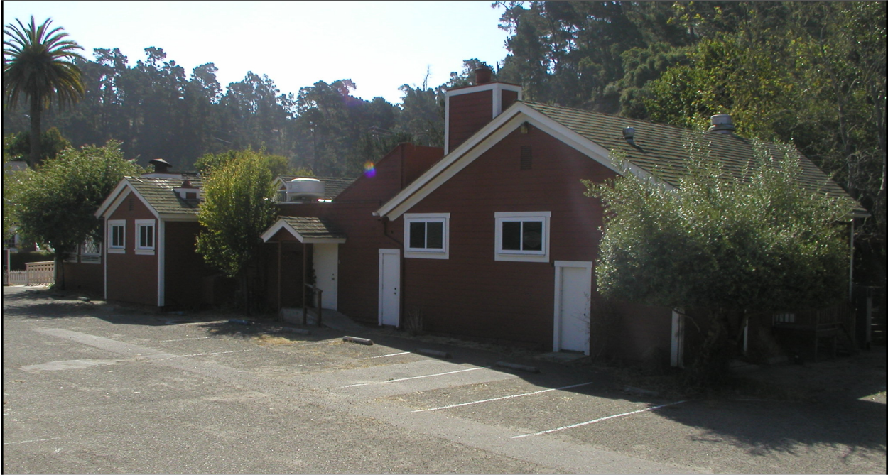
Figure 14: North Facade (August 2012)
