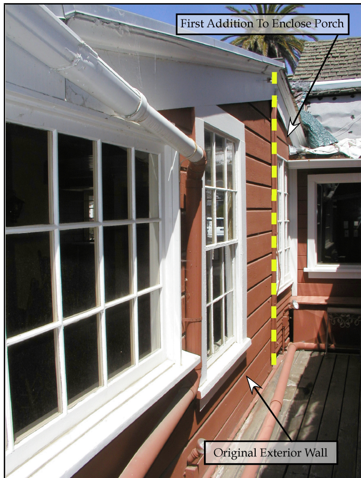
Figure 22: Original Exterior Wall Facing Enclosed Open Area (August 2012)
