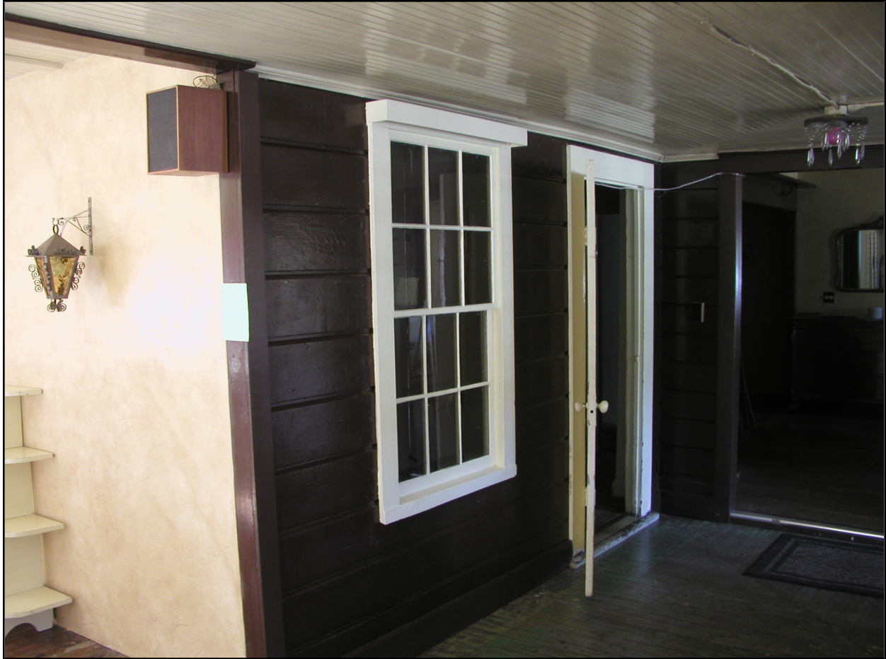
Figure 18: Original Exterior Wall Now Interior (August 2012)
