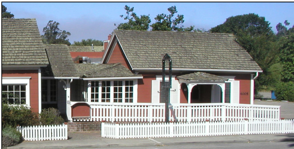
Figure 19: New Front Entrance With Ramp (August 2012)
