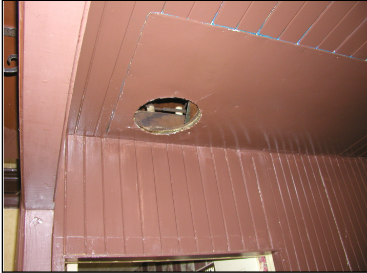
Figure 21: Original Chimney Hole & Wall Sheathing (August 2012)
