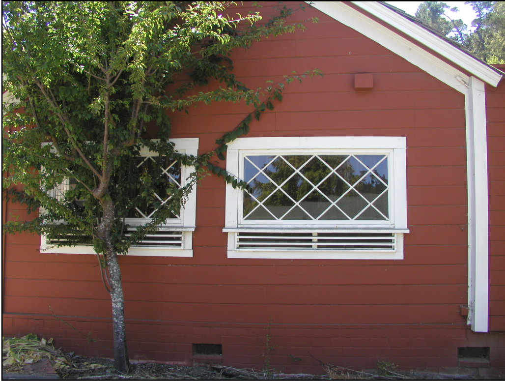
Figure 23: Vents Below Windows On North Facade (August 2012)
