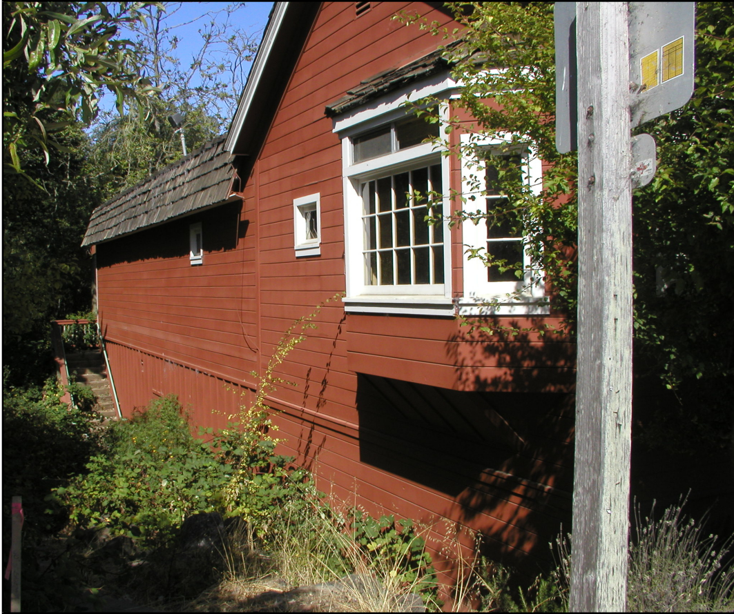
Figure 16: South Facade (August 2012)
