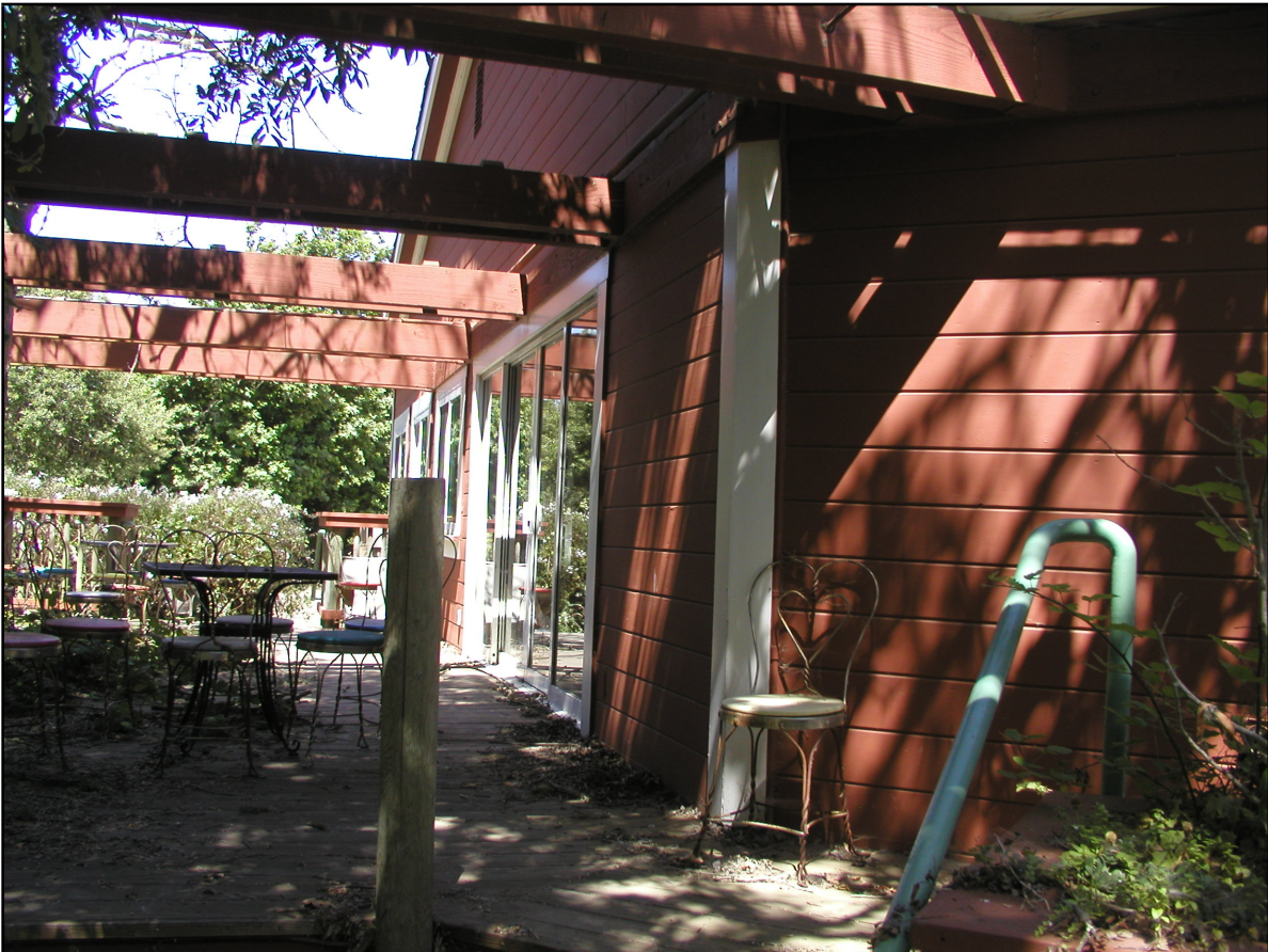
Figure 15: Portion of West Facade (August 2012)
