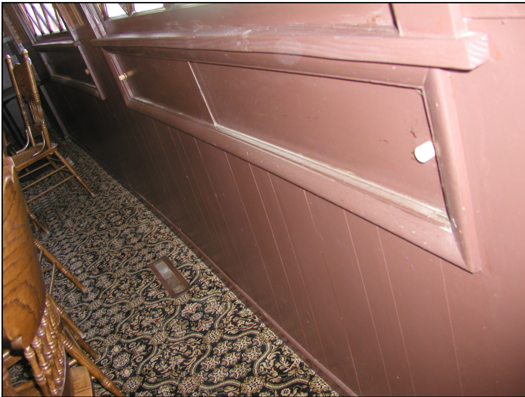
Figure 24: Interior Access To Same Vents (August 2012)
