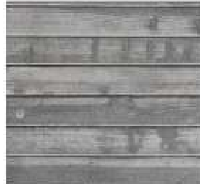
Board formed concrete at planters
