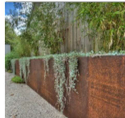
COR-TEN Planter and Conc Retaining Wall
